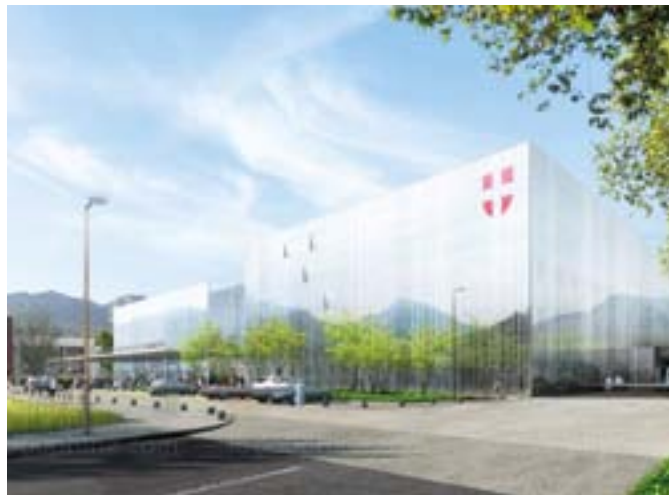
Chambery Hospital - Chambéry (France)
